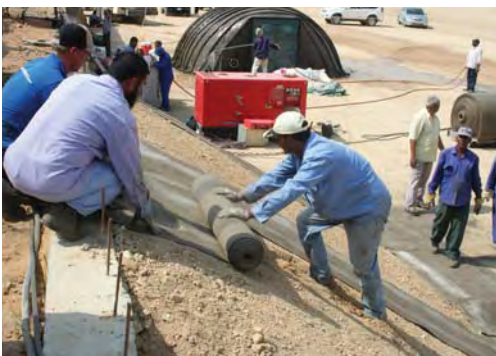
Short lengths of CC can be provided in man portable lengths for manual application.
