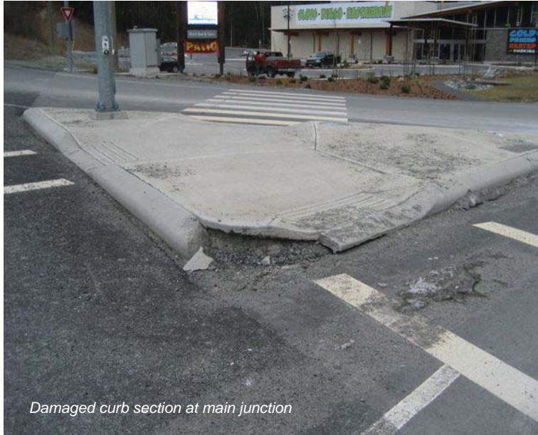
Damaged curb section detail
